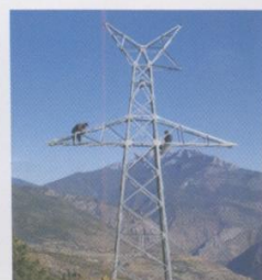
(C)35kV线路铁塔组立
